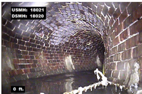
Brick storm sewer pipe
